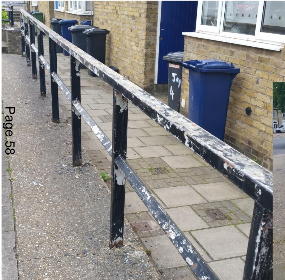
St Matthews Street area before and after work undertaken by City Rangers and Community Payback
